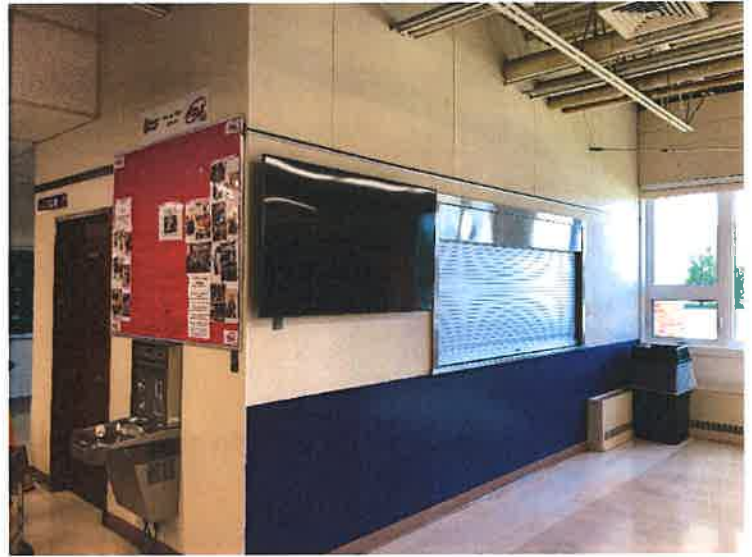
Concession stand counter is not handicap accessible
