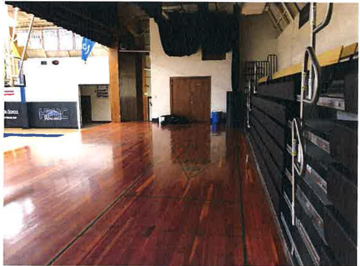
Missing fall protection (guard railing) at stage front when bleachers are used
