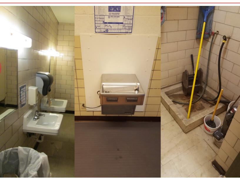
Corrective Action: Janitor's closet mop sink does not meet current codes. Replacement of faucets is required and vacuum breaker needs to be added. Drinking fountain is not ADA compliant and need to be replaced. Given the age of the building, the domestic water piping should be replaced throughout.
