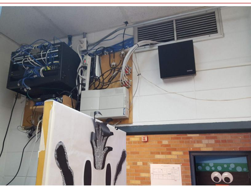
Corrective Action: Data room is not properly temperature controlled. Auxiliary cooling unit would need to be added. Cabling through existing ventilation system needs to be rerouted.
