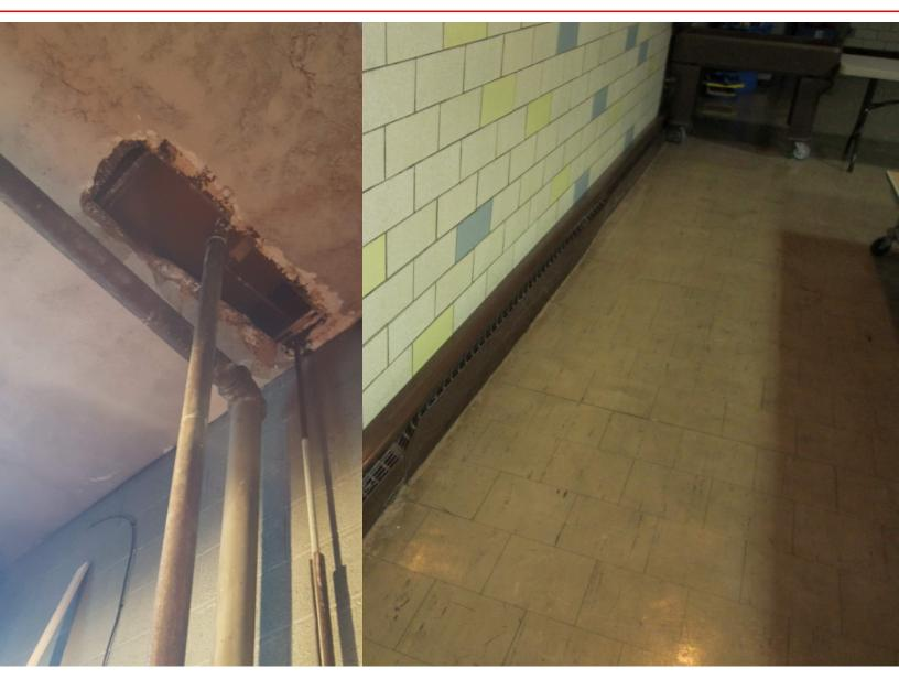
Corrective Action: The flooring, most plaster walls, pipe insulation and other components of the building contain asbestos and would require abatement prior to any new construction or renovation.
