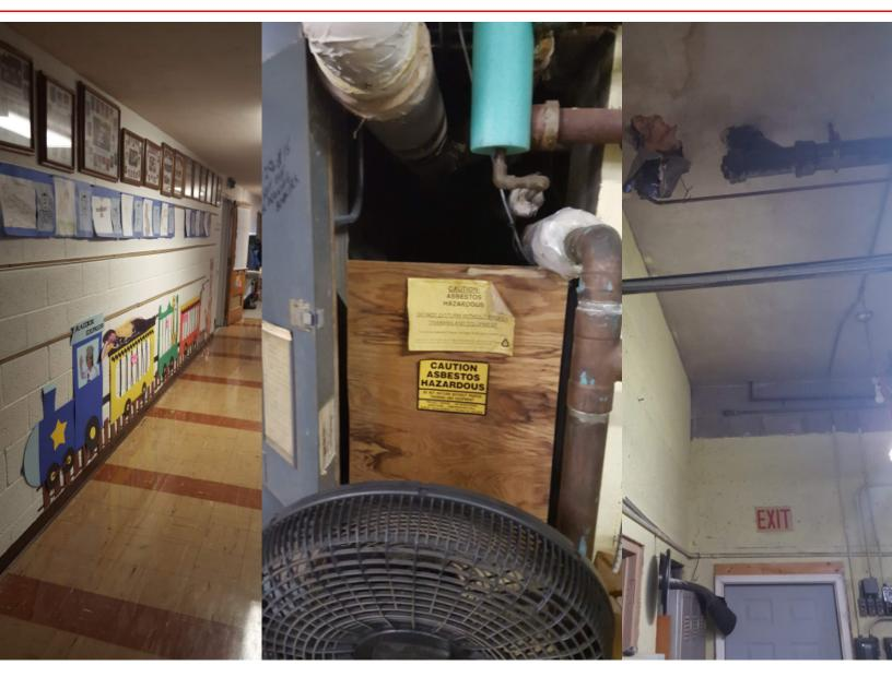
Corrective Action: The flooring, most plaster walls and ceilings, pipe insulation and other components of the building contain asbestos and would require abatement prior to any new construction or renovation.
