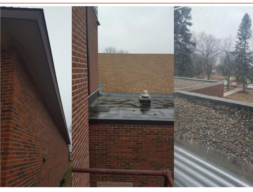
Corrective Action: Exterior walls, roof and windows of entire building provide poor insulation and should be corrected to provide a comfortable and efficient environment. All exterior walls will be required to be furred out to add insulation. All roofs will require added insulation and repair. Install gutters and downspouts on gymnasium roof to protect foundation from seepage and reduce erosion.
