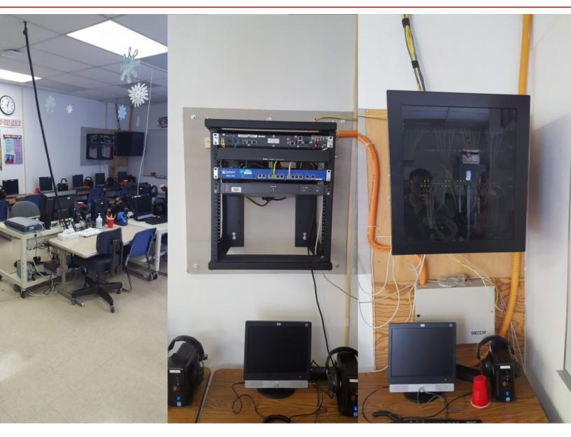
Corrective Action: Data room / computer classroom is not properly temperature controlled. Auxiliary cooling unit would need to be added.
