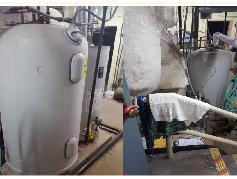
Corrective Action: There are both an electric water heater and a gas water heater. Both water heaters are approaching the end of their useful life. The electric water heater is the newer of the two and was installed in 2001.
