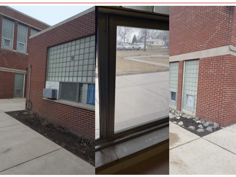
Corrective Action: Exterior walls, roof and windows of entire building provide poor insulation and should be corrected to provide a comfortable and efficient environment. All windows are single pane or glass block and are in need of replacement.
